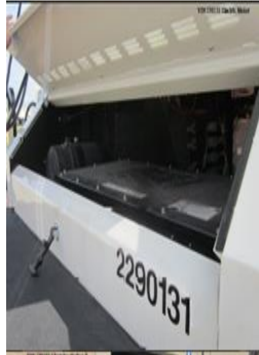
Terminal Tractor Electrical Component Compartment
