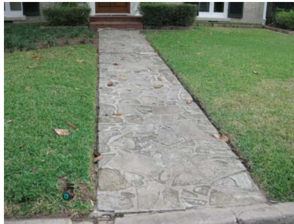
Figure 5.4. Cut stone with an appropriately abrasive finish.
