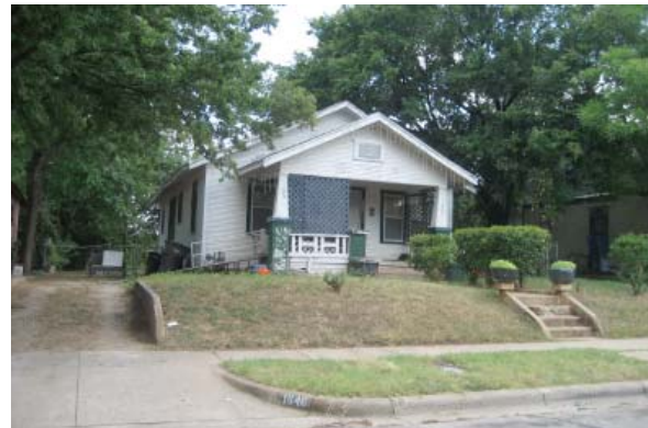
Figure 6. Interior lot condition.
