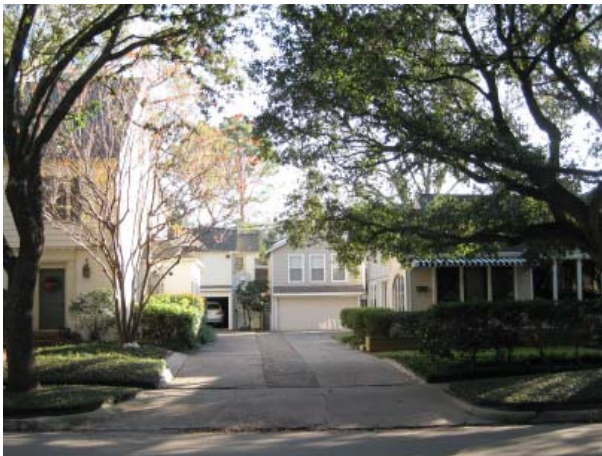
Figure 2.7. Garage apartments situated above detached garages.
