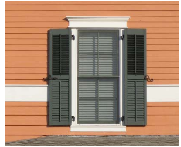
Figure 4.13. Shutters, when used, shall be real and operable components of the window treatments.
