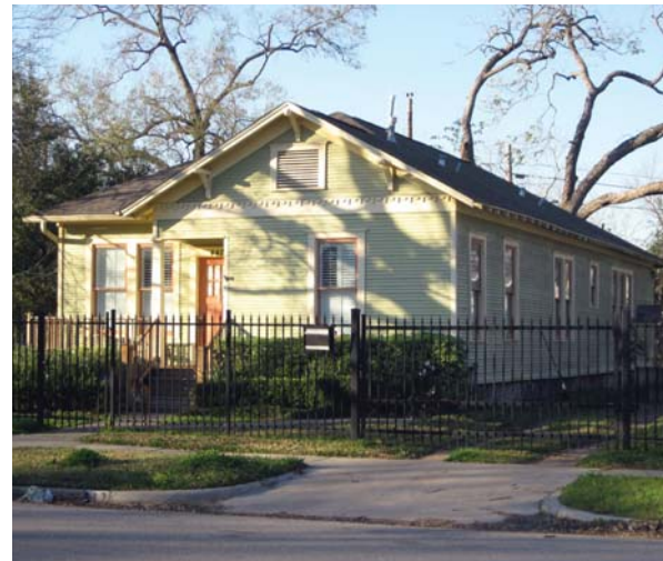
Figure 4.18. Exposed rafter tails and roof overhangs.
