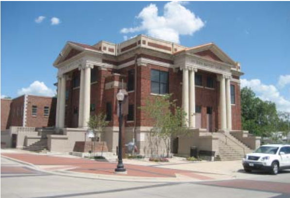
Figure 2.11. Church on southeast corner of Evans & Verbena.
