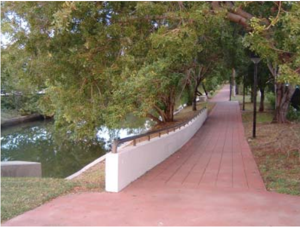
Figure 5.1. Concrete with integral color tone and stamped patterned concrete.
