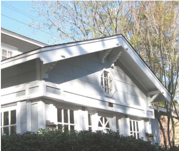
Figure 4.14. Specialty windows shall be used sparingly as accent pieces, and only if compatible with building style.
