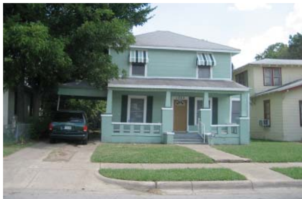
Figure 5. Interior lot condition.
