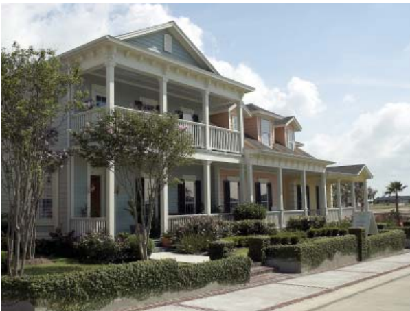
Figure 5.3. Plain concrete arranged in panels framed by brick.
