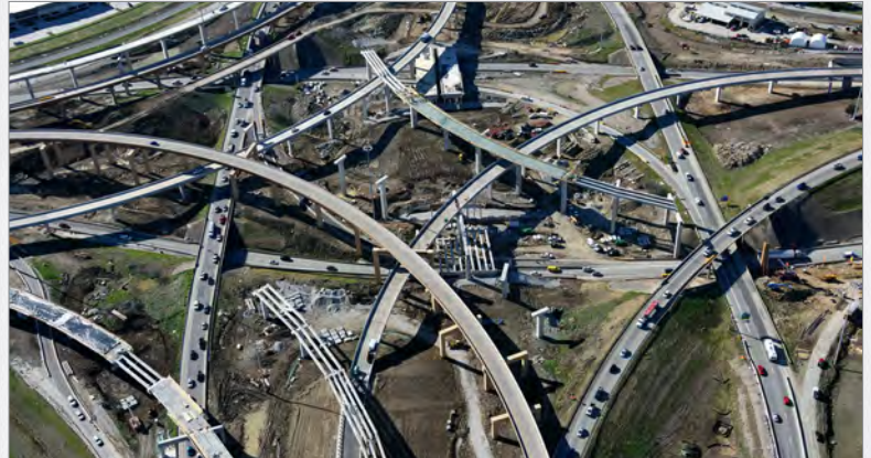
Feb. 2016 - I-35W/I-820 Interchange Looking South
