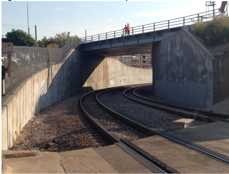
Figure 3: 7 th Street Railroad Underpass
