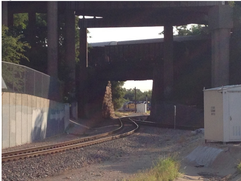
Figure 4: “The Hole in the Wall”
