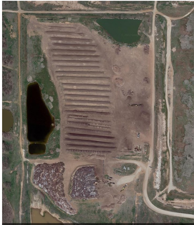
Figure 1 City of Wichita Falls Compost Facility
