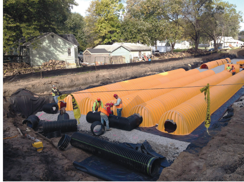
Soakage Trench installation. (Source: Wikipedia, CC BY-SA 3.0)
