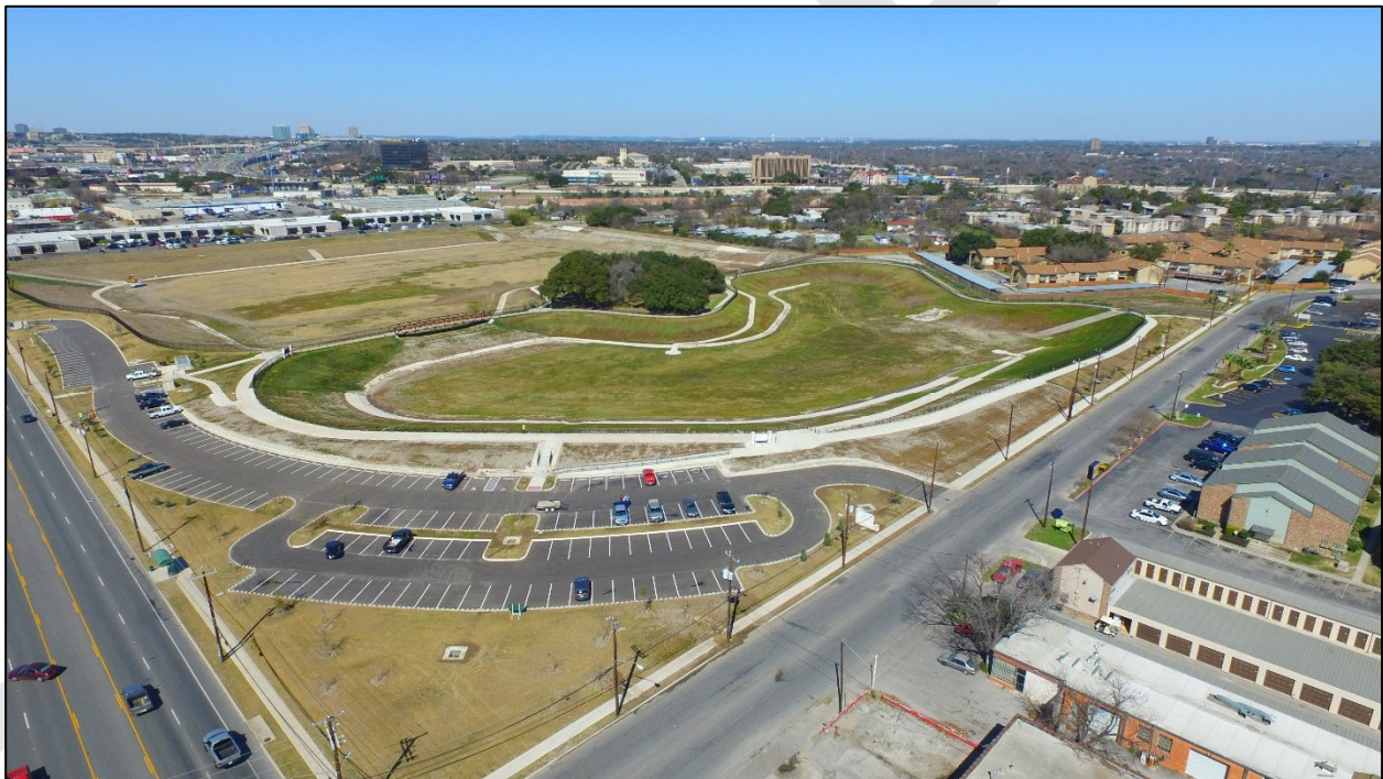
Figure 1. Laddie Place Phase III Regional Storm Water Facility resulted from a combined effort of Bexar County, the City of San Antonio and the San Antonio River Authority to convert a 28.5-acre shopping center that was almost entirely covered by impermeable surfaces except for heritage oak trees. The heritage trees are a defining feature of the former shopping mall that was converted to a regional detention facility and park with natural elements that improve the stormwater quality and increase stormwater volume.
