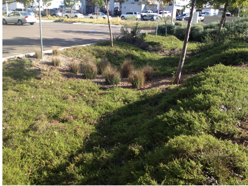
Enhanced Swale in San Diego, CA. (Source: Tetra Tech)
