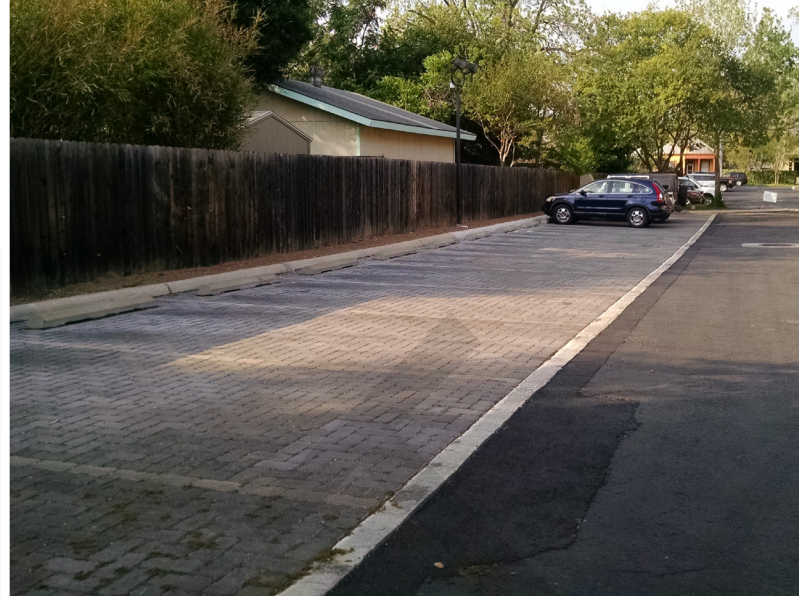
Permeable Pavement in San Antonio, TX. (Source: Tetra Tech)
