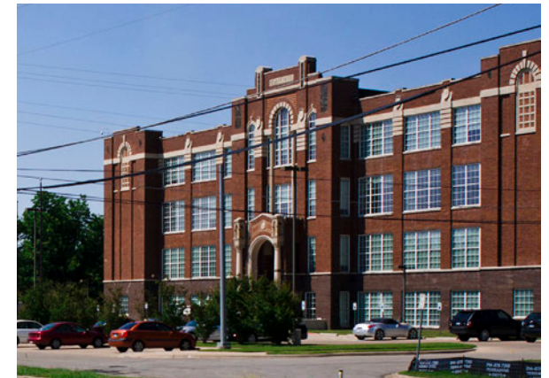
The Guinn Justice Center is located in the repurposed High School building that was constructed in the early 1900s.
