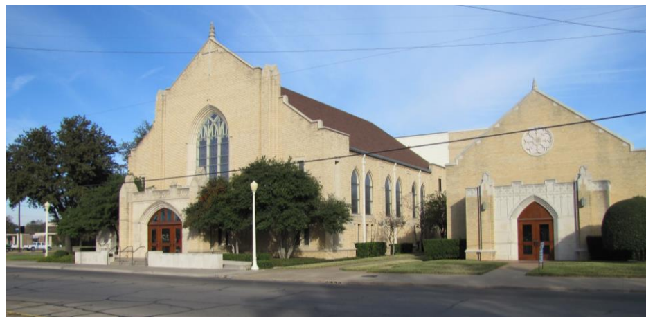
First Baptist Church on Brown Street
