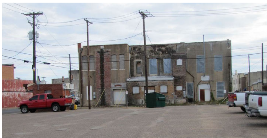
Back of building along the alley opposite from the small cafe
