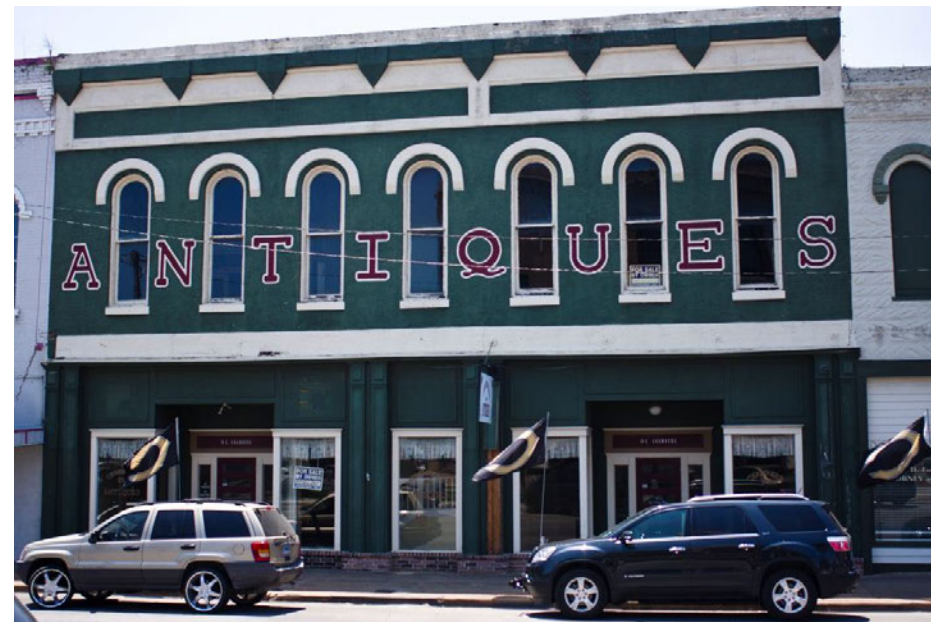
Two story building façade along Henderson between Caddo and Main Streets
