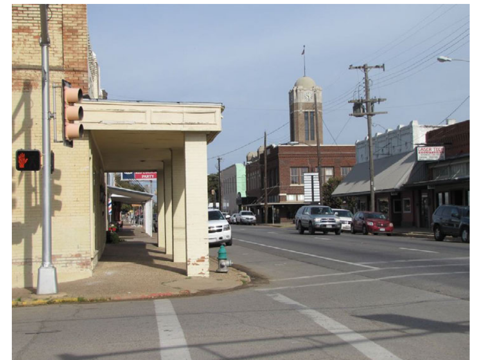
Corner of Harrell Street and Main Street (SH171)
