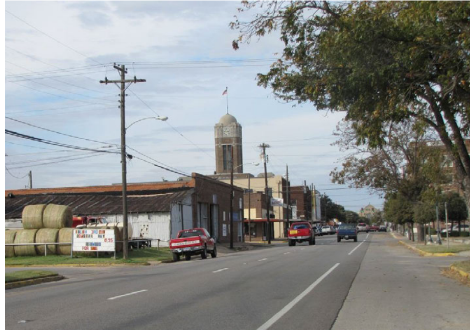
View north along Caddo Street (SH171)
