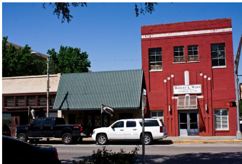
Building facades on Main Street (SH171) between Henderson and Caddo Streets
