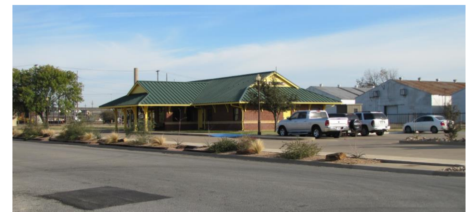
Intermodal station along Border and Wardville Streets
