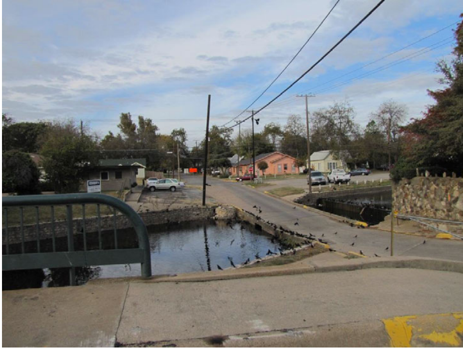
Buffalo Creek at Henderson Street where Buffalo Street crosses the creek
