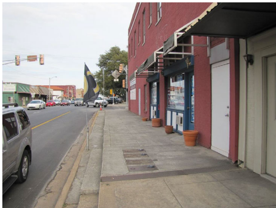
Stepped and raised sidewalk along Henderson Street (SH67)
