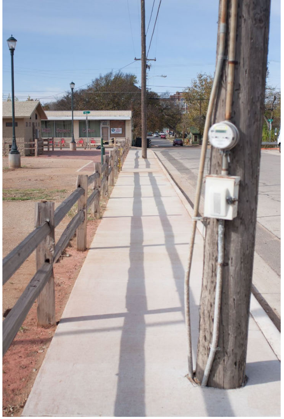
The location of utility poles in this new sidewalk impacts its aesthetic character and makes it more challenging for people in wheel chairs or couples walking abreast. Location: Harrell Street along Market Square.
