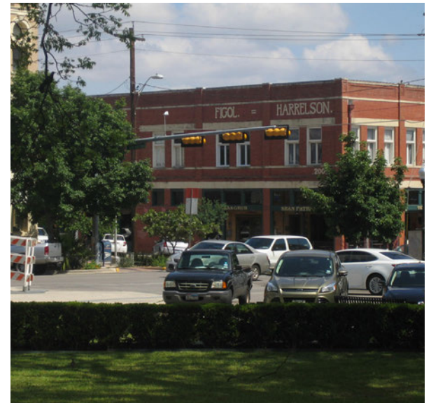
Shops around Courthouse Downtown
