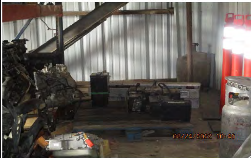
Batteries stored off ground and under cover.
