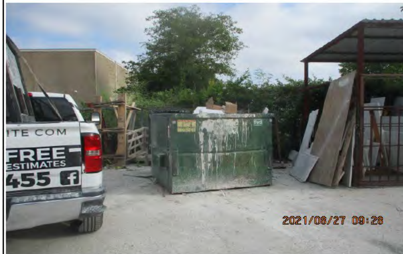
Dumpster must be closed
