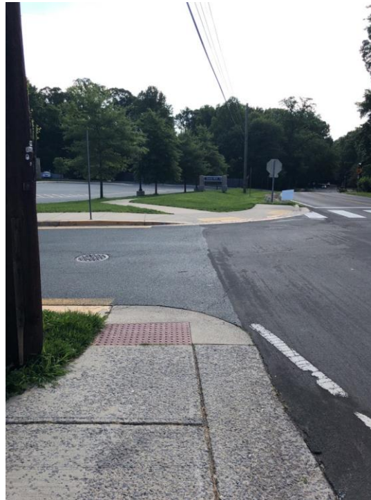
6. Missing crosswalk and awkward intersection design at Bells Mill Rd and Democracy Ln
