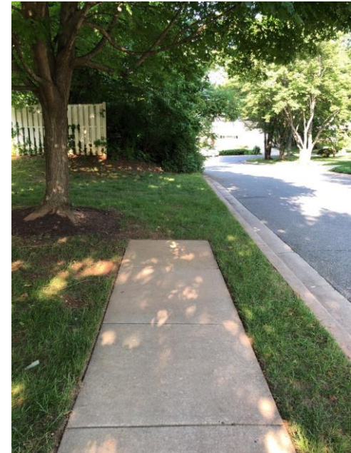
13. The sidewalk on Larkmeade Ln terminates just prior to the athletic field path. Tree is within County ROW.
