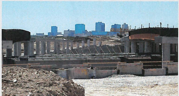
Future I-35W Lanes at Railroad Crossing near Long Avenue
