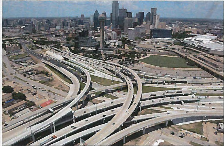
Pictured above: An aerial view looking toward downtown Dallas at the newly reconstructed Mixmaster now carrying more than 450,000 vehicles each weekday.
