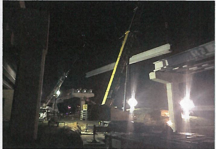
SH 121/360 interchange construction
