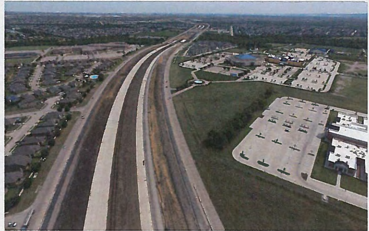
Concrete paving for the new mainlanes near Debbie Lane
