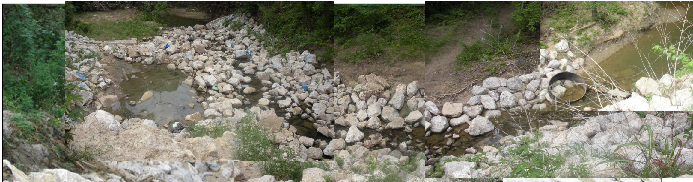
At 96" RCP Outfall near Christopher Drive
