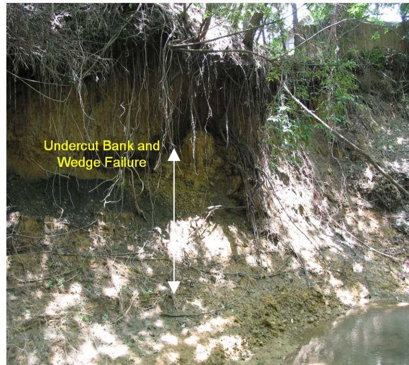
Toe Failures
