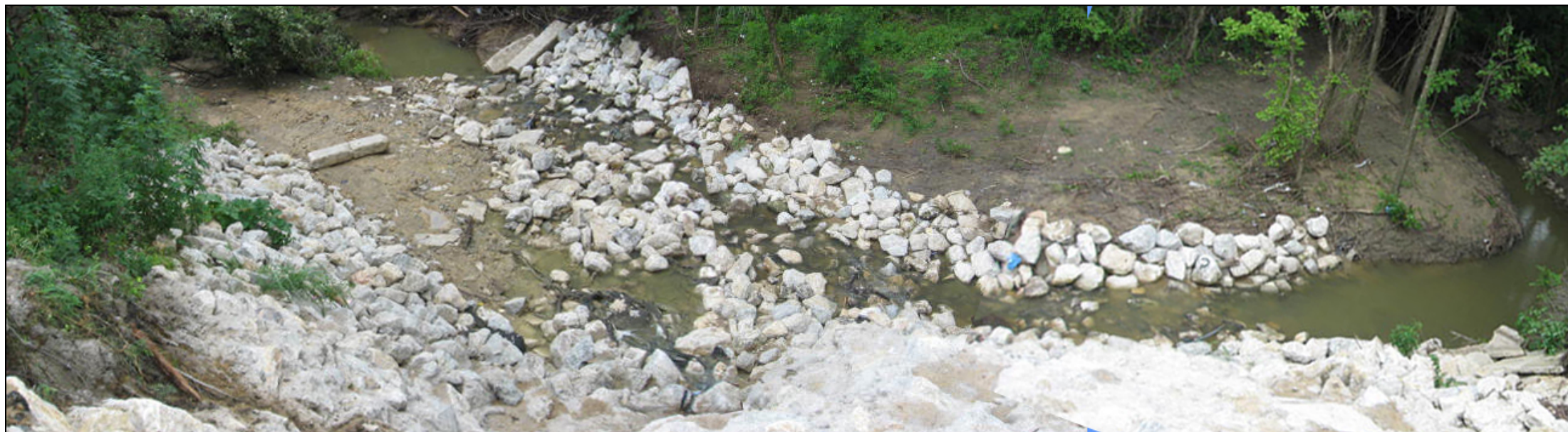
At 96" RCP Outfall near Christopher Drive
