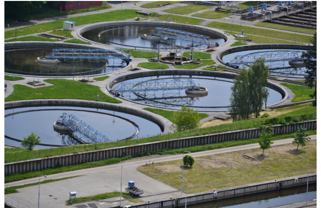
Wastewater treatment plant; Photo courtesy of fotolia
