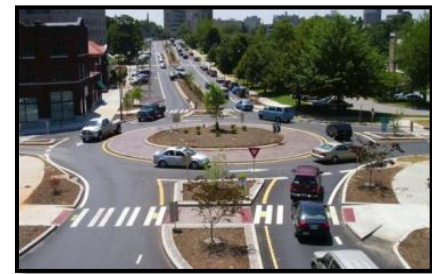
Figure 47: Example of Modern Roundabout
