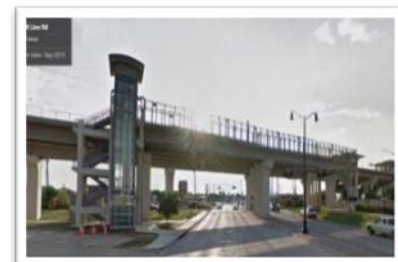
Figure 17: Downtown Carrollton DART Station platform extending over Belt Line Road with a stair and elevator tower on the opposite side of the roadway from the DART station
