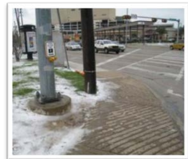
Figure 23: Pedestrian Push Buttons and curb ramp
