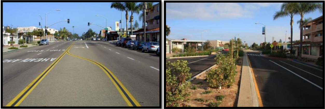
Figure 44: Example of before and after complete streets design which balance the needs of pedestrians, bicyclists, transit, and motor vehicles
