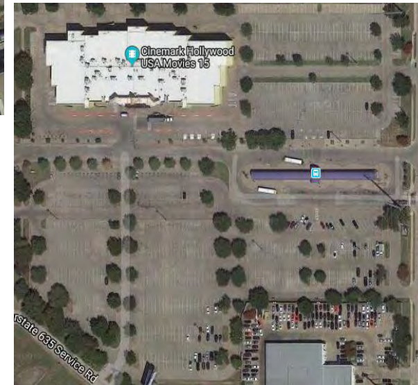
South Garland Bus Transit Center
