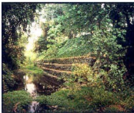
Figure 3.22 Gabion Baskets Installed for Slope Stabilization along a Stream
