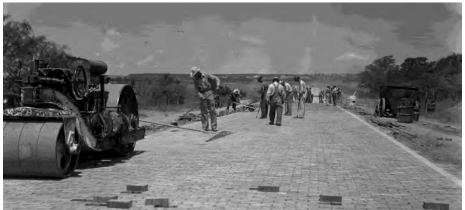
1938: workers put the finishing touches on the original brick of SH 1/Bankhead Highway between Weatherford and Mineral Wells, which later became U.S. 180.
