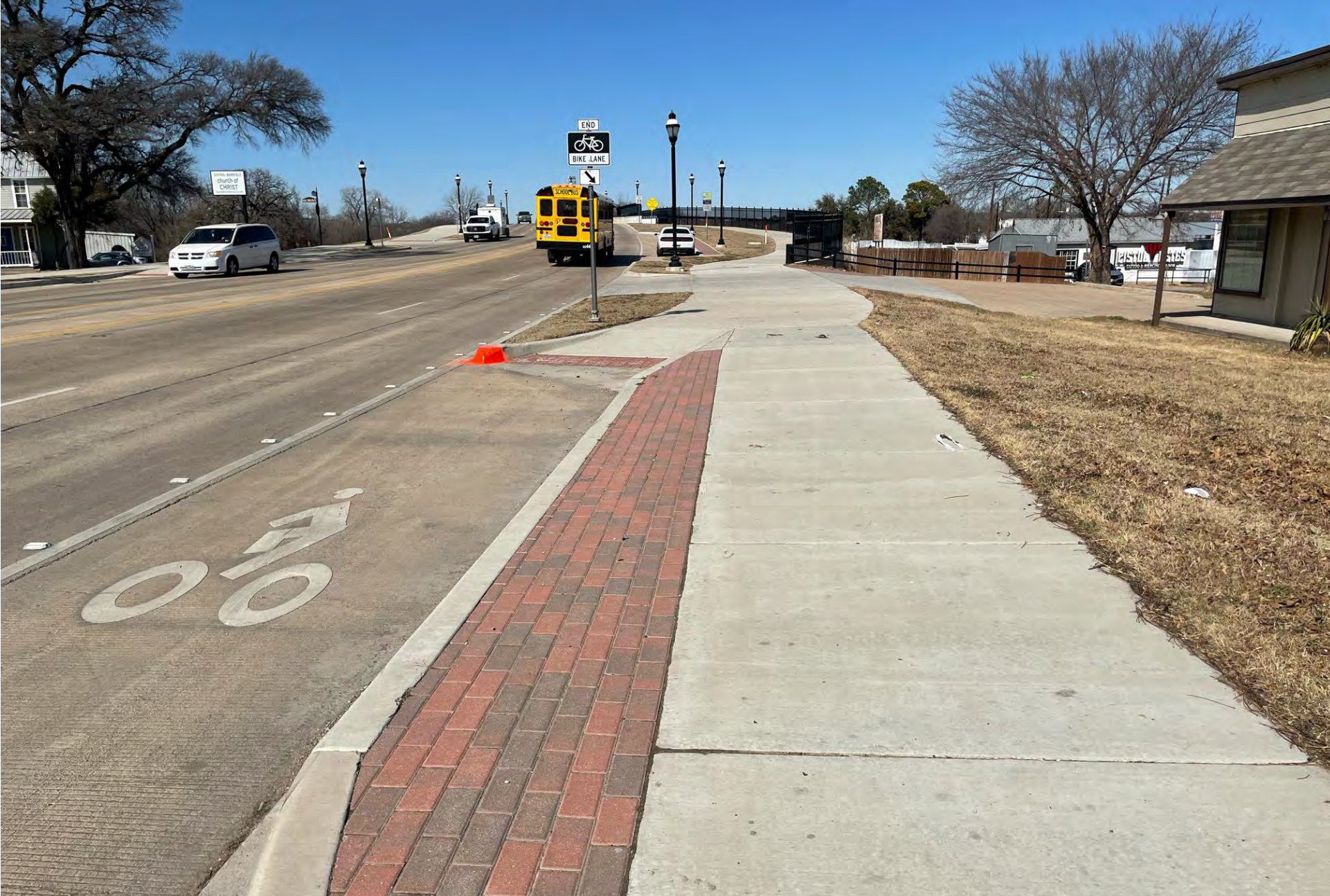
North Bound Bike Lane Transition to the shared use path
