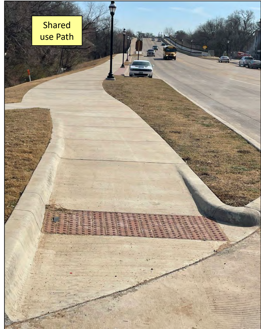
North Bound Bike Lane Transition from the shared use path to the Street
