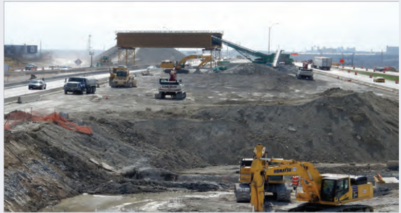
March 2017 - I-35W construction at 28th Street
