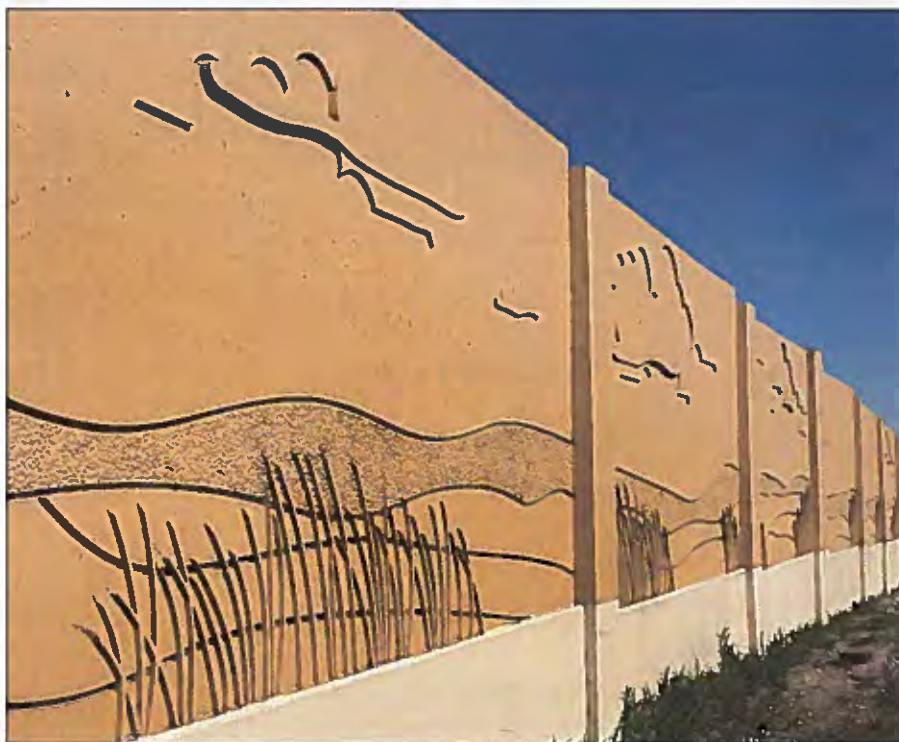
Decorative noise barrier near the intersection of Allen Drive has a carved relief representation of the Blacklands Prairie, giving it a unique and attractive appearance.
