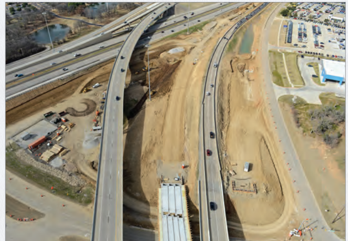
SH 121/360 interchange construction
