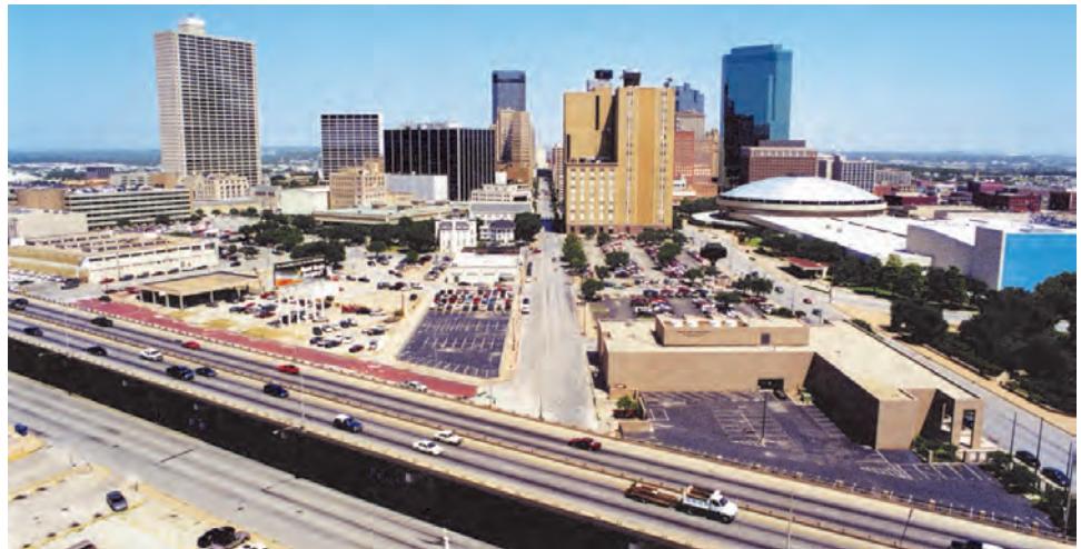
Leading into the Mixmaster, the I-30 elevated expressway was a landmark in the city skyline for 40 years until it was removed in 2001 to allow for the development of Lancaster Avenue and southern downtown Fort Worth.
