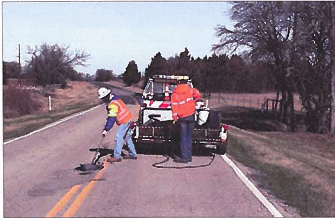
Maintenance crew patches a road in Navarro County.
