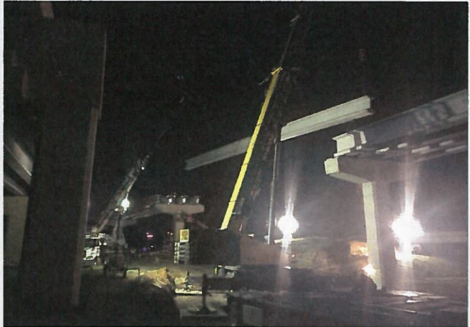
SH 121/360 interchange construction
