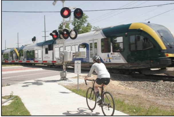
Existing DCTA Rail Trail shared use path along the A-train rail corridor in Denton, north of the TIGER project area.
