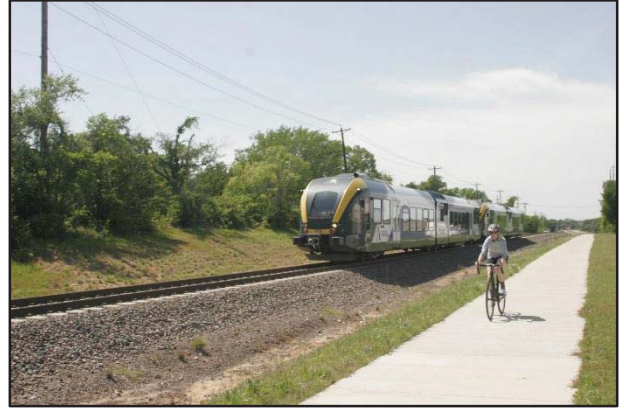
Existing DCTA Rail Trail shared use path along the A-train rail corridor.
