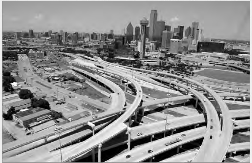
Pictured above: An aerial view of the Horseshoe Project looking east toward downtown Dallas of the new I-30/I-35E interchange.
