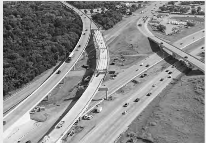
SH 121/360 interchange construction
