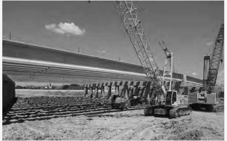
Future SH 360 bridge at Camp Wisdom Road
