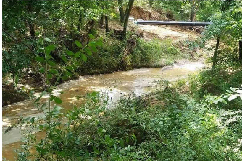
❖ Water main break
