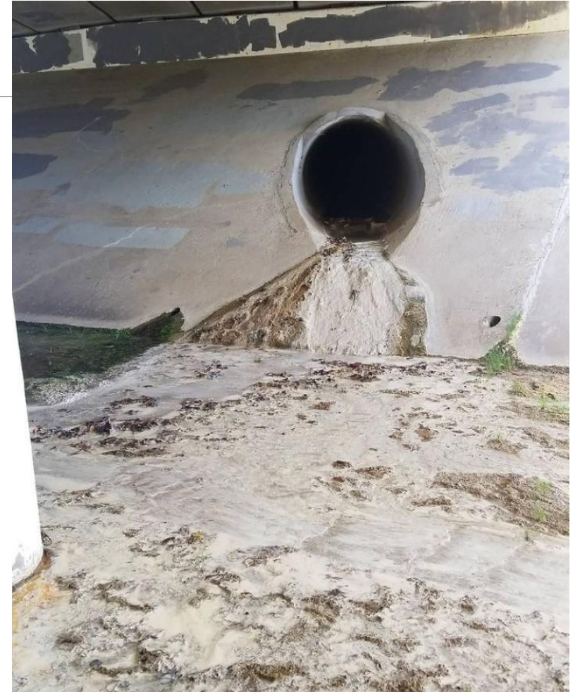
The pH of this discharge was ~12.0! Temperature was also warmer than expected! Upstream activity was stopped immediately
