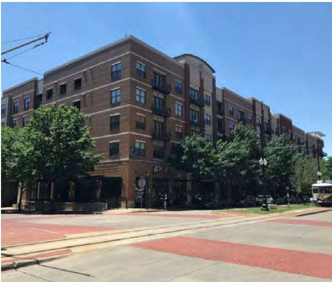
FIGURE 2.5C FLATS AT THE SAWYER (CITYPLACE/UPTOWN STATION)
