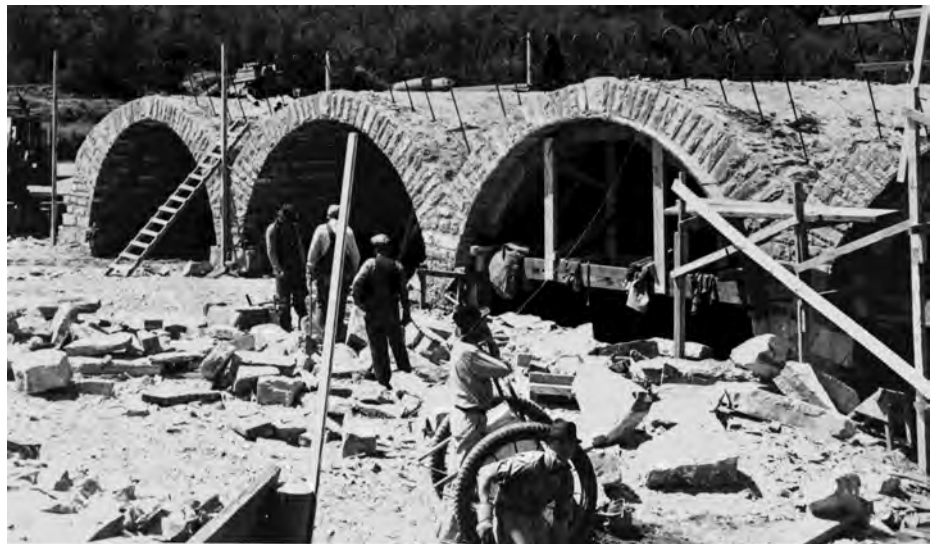
The SH 16 arch masonry bridge at the Possum Kingdom dam in Palo Pinto County. Designed by the Fort Worth District and built by the Works Programs Administration (WPA) in the 1930s, this beautiful bridge is still in use over 80 years later.
