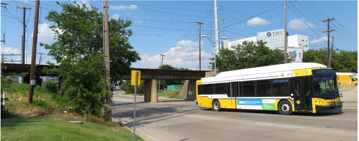
Figure 2: Component A1, Inwood Bridge
