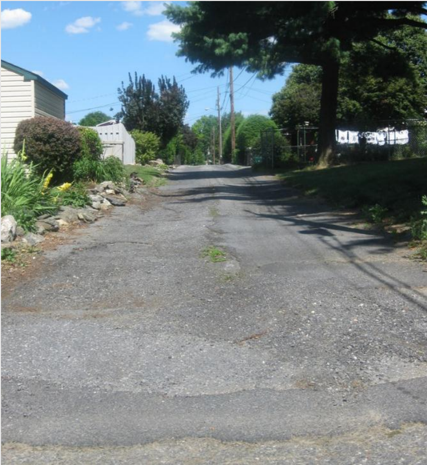
Conventional reconstruction (8-inch reinforced concrete) ~$20.30/SF
