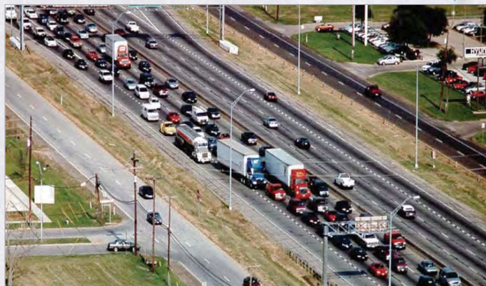
State Highway 183 Corridor
