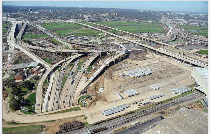
Looking west/southwest at the downtown Dallas mixmaster. Interstate I-30 on the right, I-35E on the left.
