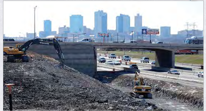
Feb. 2015 -- Expansion work on I-35W at 28th Street.
