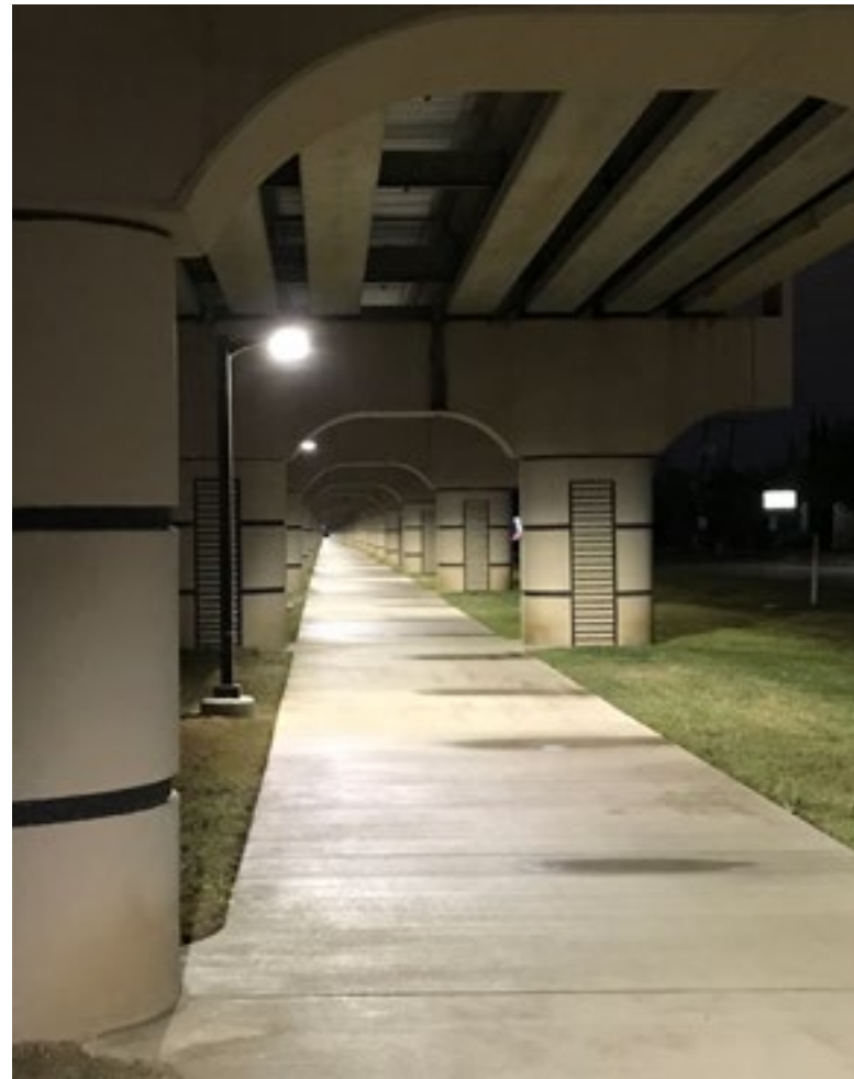
Existing Rock Island Road Sidepath lighting
