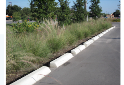
Bioretention Facility in San Antonio, TX. Source: Tetra Tech
