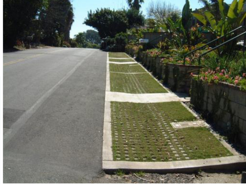
Modular Porous Paver System in Encinitas, CA. (Source: Tetra Tech)
