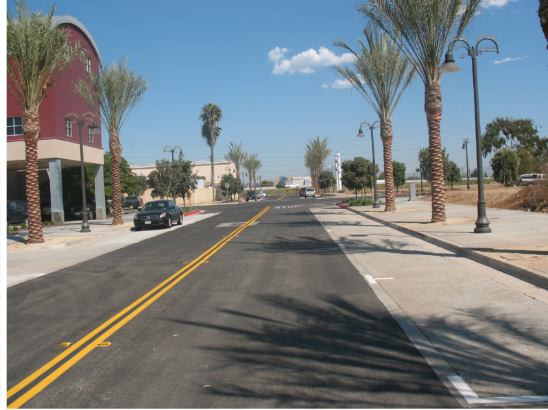
Porous Concrete in San Diego, CA. (Source: Tetra Tech)
