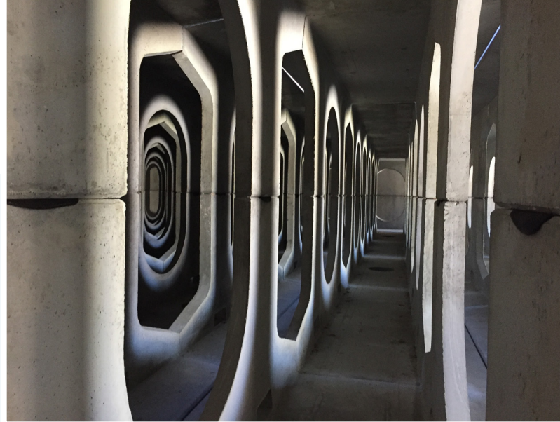
Underground Detention Facility in Los Angeles, CA. (Source: Tetra Tech)
