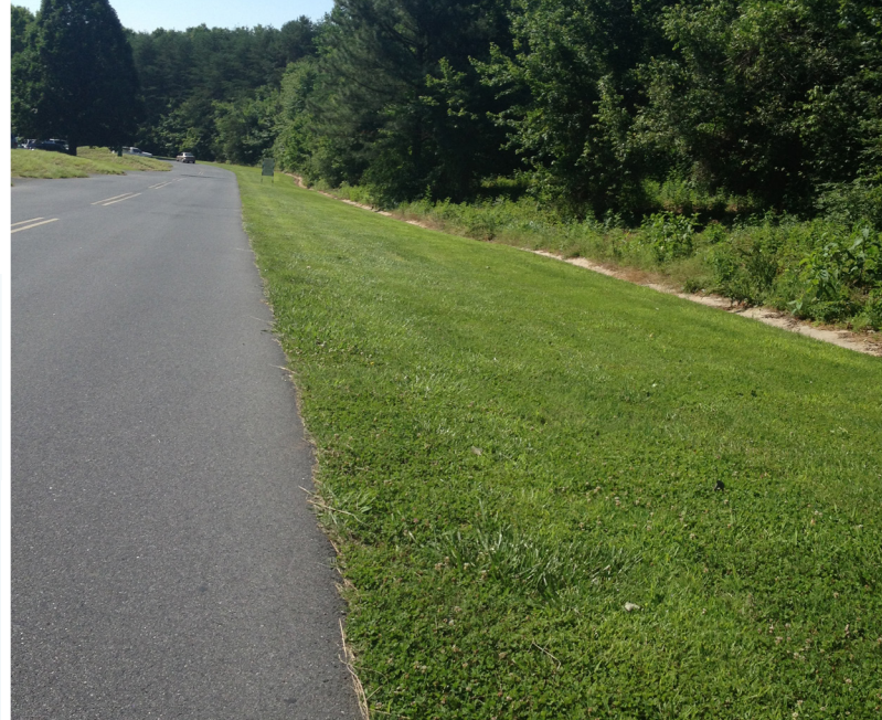
Filter Strip in Asheboro, NC. (Source: Tetra Tech)
