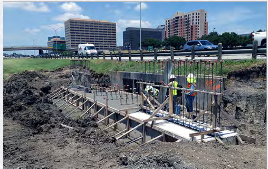
Start of construction on State Highway 114.
