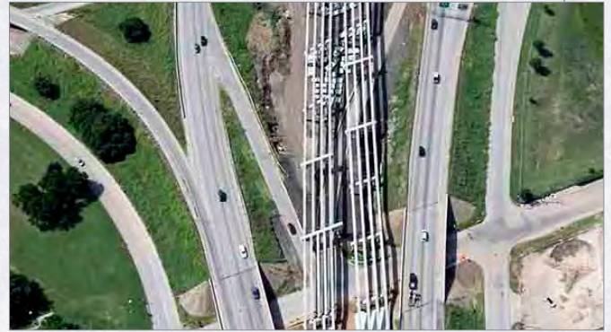
July 2015 -- I-35W from Pharr St. to SH 121 looking north.
