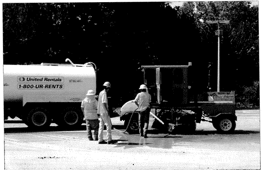
From Left: Bobby Hale, Brian McCarthy and Randy Germany of TxDOT's Denton Area Office work with the Texas Department of Parks and Wildlife to remove 1,110 tons of sand and dirt pushed into the Greenbelt Corridor of Ray Roberts Lake State Park by flood waters this past summer.
